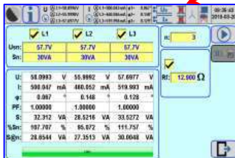
PT burden test
